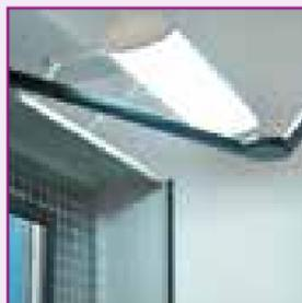
Lighting of the space between units. The illumination is controlled electronically and works only above the unit currently used by a personnel. Lighting covers are placed on metal trusses, screwed to the top shelves (the covering). The illumination starts automatically when the aisle is opened and switches off when it is closed, provided software allows user to set the time after which the light switches off.
